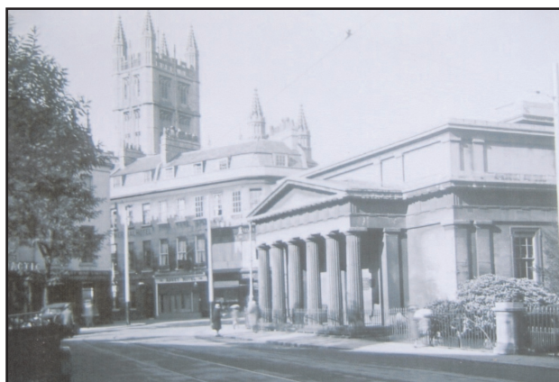
Figure 4. BRLSI, original building at Terrace Walks, Bath. Image courtesy of Matt Williams and the BRLSI.
