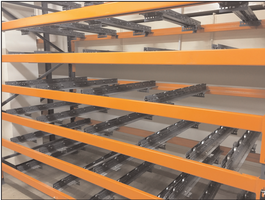
Figure 3. The old racking, just prior to its removal in spring 2017.
