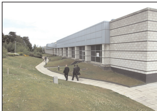
Figure 4. Swords CRC is a former electronic factory, seen here from the front.
