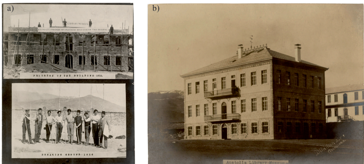
Figure 2. A) Construction phases of the library-museum building in Anatolia College Merzifon. B) The final version of the museum-library building in 1914.
